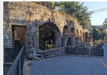
Aqueduct Cal Pla
